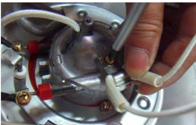
5. Fixed new fuse. (supply leads combination)
